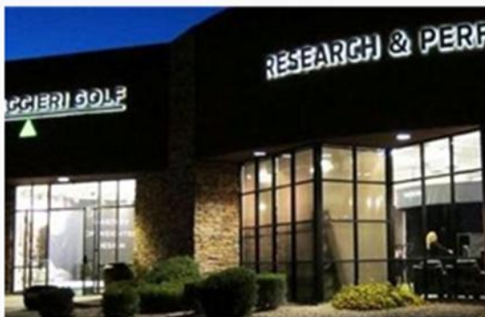
PIPELINE: Linthicum has completed construction on Bocchieri Golf's new "digs" in the Airpark
